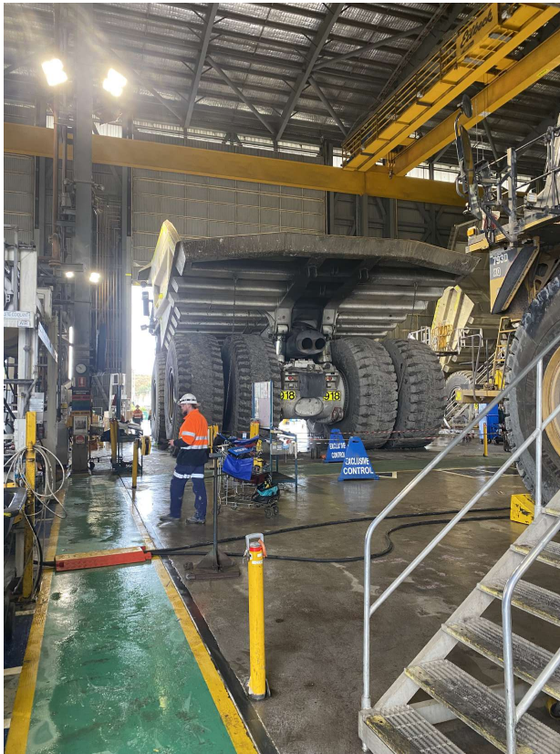
Figure 3.5 – Haul Truck Workshop at MAC
